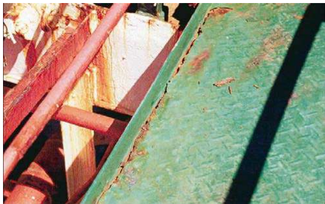
Catwalk cracked.
