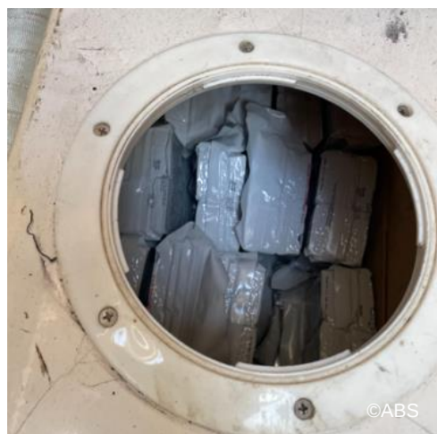
Missing lifeboat rations replaced
