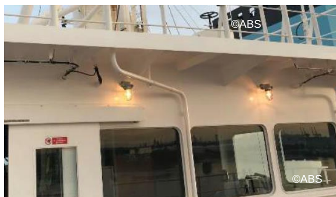
Operational test of emergency lights after repair
