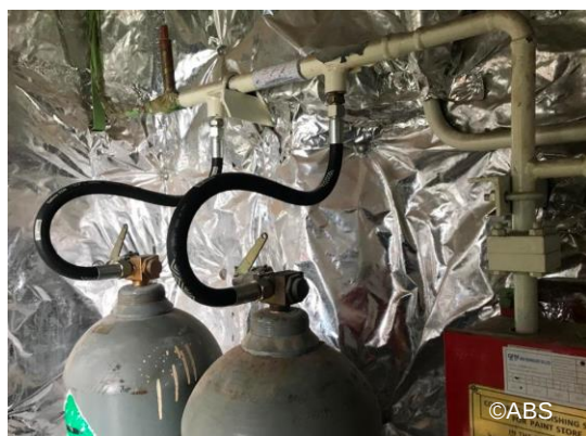
Paint store CO 2 hoses replaced
