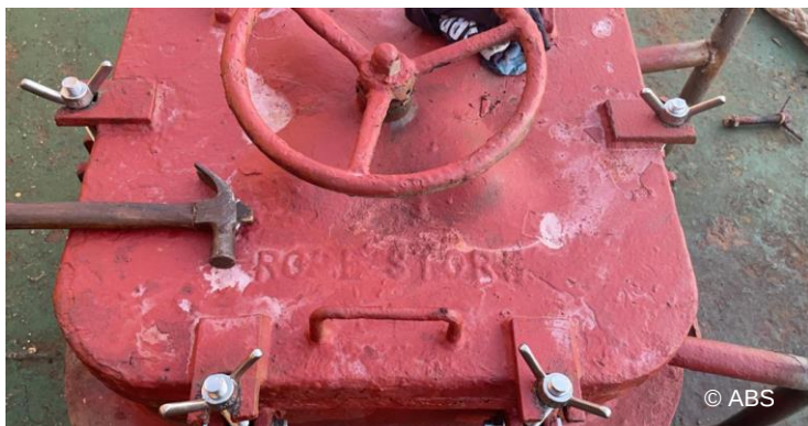
Watertight booby hatch with new dog bolts
