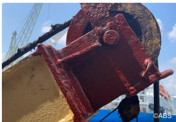
Rescue boat davit found corroded
